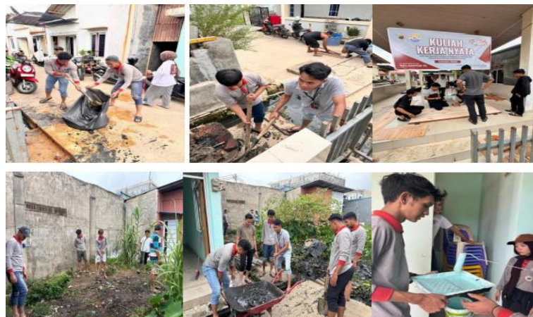
Figure 2. Process of Repairing and Cleaning Public Facilities and Drainage in RW.20/RT.02
